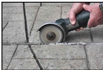
Slice through Hard or Soft Joint Sealant
