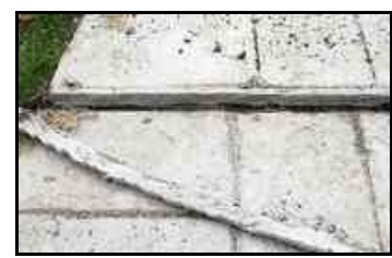
Clean, finished inside edges w one pass of the blade
